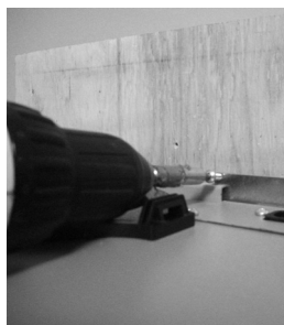
Figure 8 Secure HRV/ERV to wall-mounting bracket with the two, #8 x 3/8" screws.
