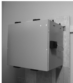
Figure 6 Hang HRV/ERV on the wall-mounting bracket.
