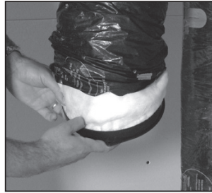
Figure 10 Insert insulation inside the double collar.
