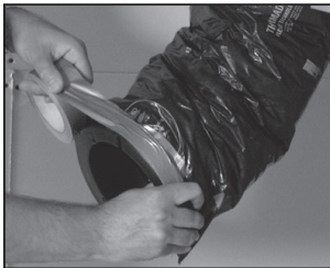
Figure 11 Finish by taping the vapor barrier to the collar to ensure proper seal.
